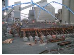
1800 m 3 Raft Slab – Lafarge Silo Foundation
