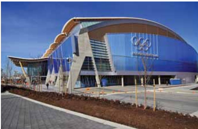
Exterior view of the Richmond Olympic Oval (Photo courtesy of Rempel Bros. Concrete Ltd.)
