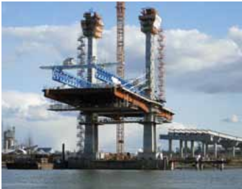
Golden Ears Bridge deck construction over the Fraser River, March 2008
