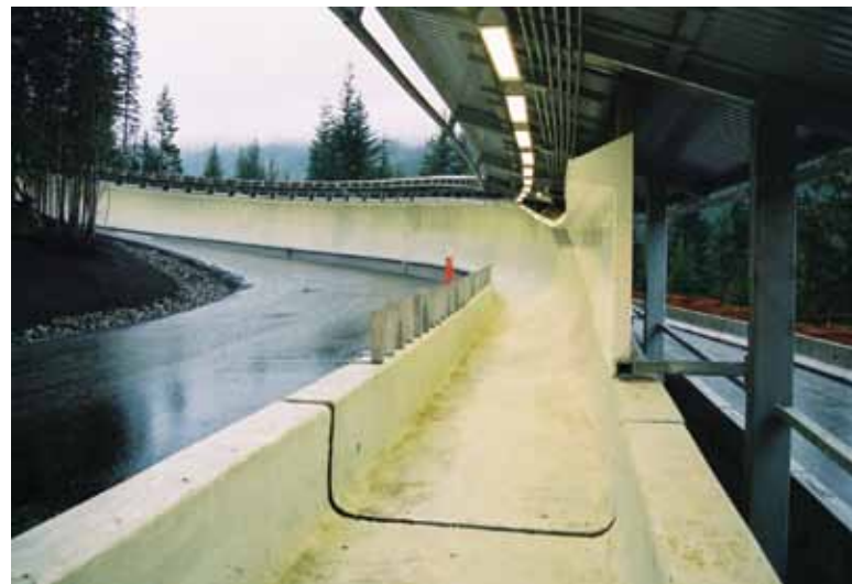
Closeup of the concrete sliding track (Photo courtesy of Stantec)
