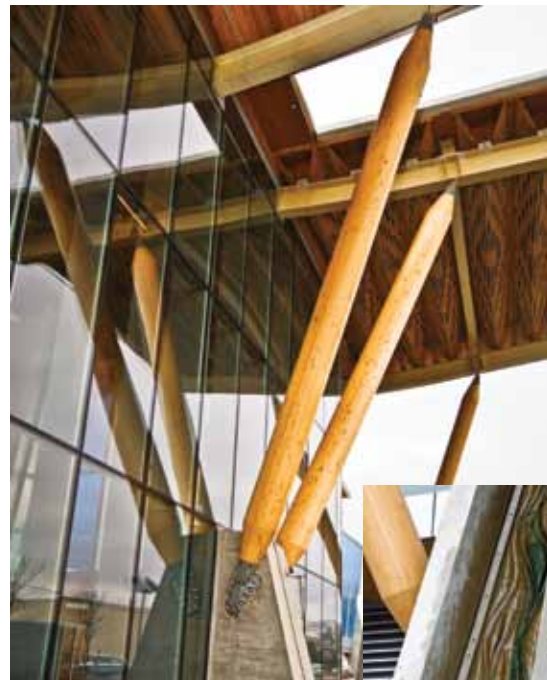
Buttresses supporting wood struts at the Oval
