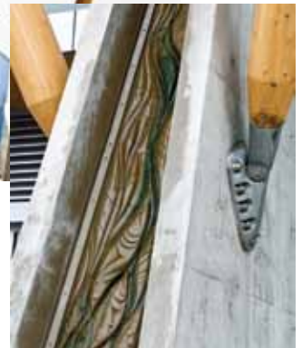
Architectural detail of runnels inset in the Oval's buttresses
