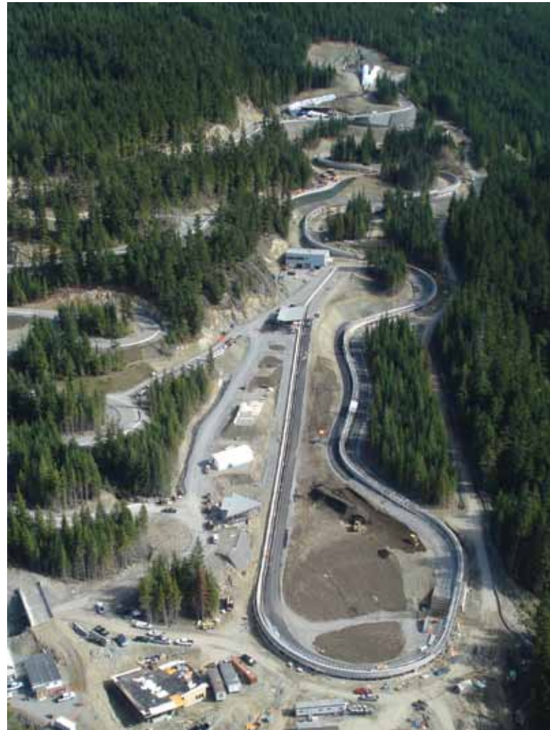
Aerial view of the concrete track at the Whistler Sliding Centre (Photo courtesy of the Vancouver Organizing Committee for the 2010 Olympic and Paralympic Winter Games)
