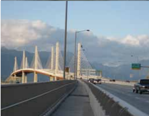
Golden Ears Bridge as seen from the south approach, October 2009 (Photos courtesy of LVM-JEGEL)
