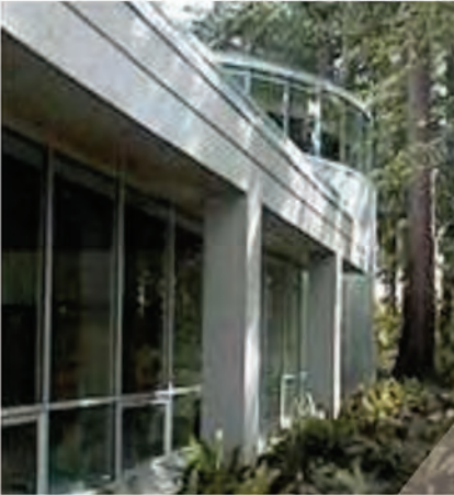
University of British Columbia's Liu Centre for Global Issues is constructed with recycled materials including high volume Fly Ash concrete.
