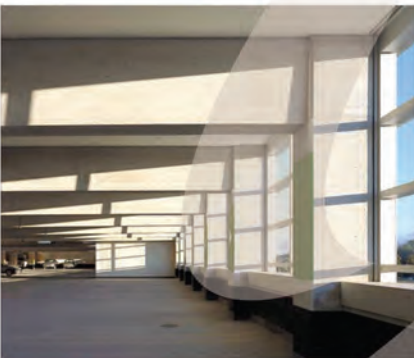
The fine, durable finish of York University's Student Services Parking Garage is attributable to the use of high volume Fly Ash concrete. Photo courtesy of Monica Contreras.
