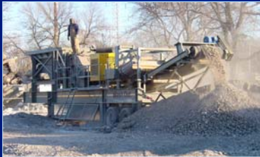
Crushing & Recycling Concrete
