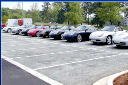
Surface parking lot paved with pervious concrete
