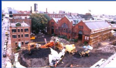
Treatment of a contaminated soil on an old industrial inner city site in Boston
