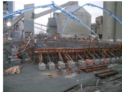
1800 m 3 Raft Slab – Lafarge Silo Foundation
