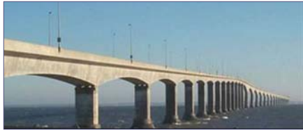
The Confederation Bridge spans 12.9 km., to link Prince Edward Island to New Brunswick mainland. Its 100-yr. design life was realized with 50% Fly Ash pre-cast concrete girders.
