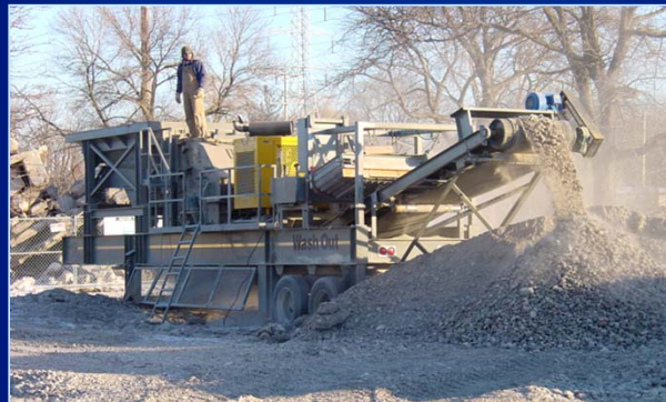
Crushing & Recycling Concrete
