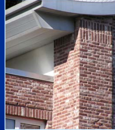
C.K. Choi Building – UBC Reused brick pavers
