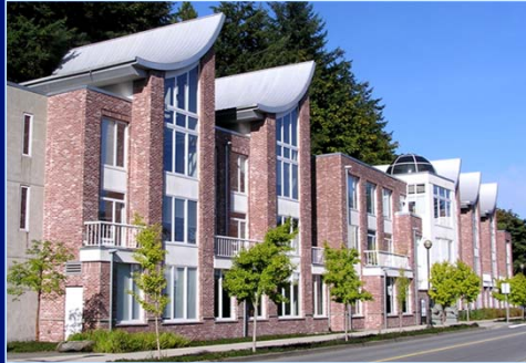
C.K. Choi Building – UBC Reused brick pavers
