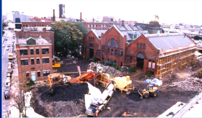
Treatment of a contaminated soil on an old industrial inner city site in Boston
